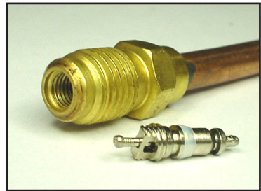
Shredder valve with core removed
